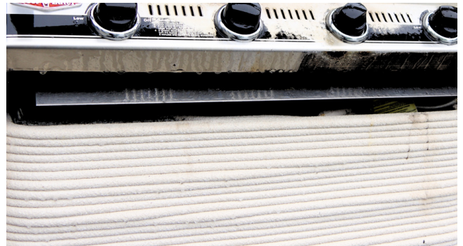
Example of grease stains on 3DPG from an outdoor grill
